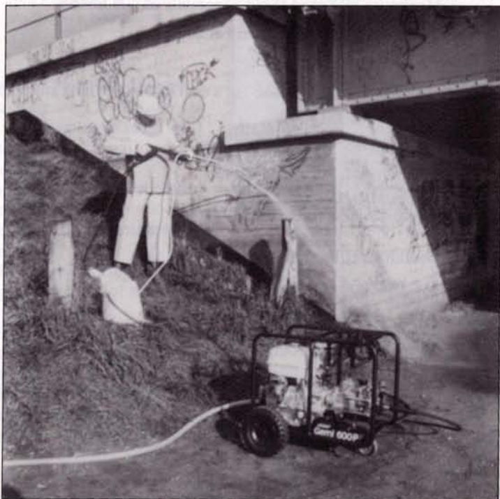
Graffiti removal using Gerni 600p with wet gritblasting attachment.
