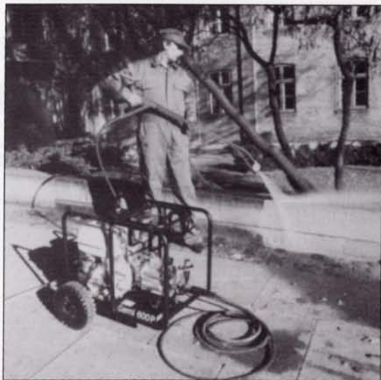
Turbo laser powered Gerni restores dirty, grimy concrete 'as new'.
