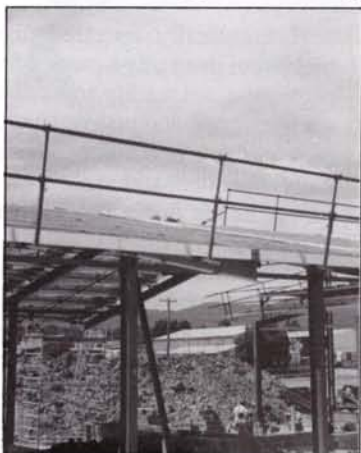
Perimeter Guardrail System.
